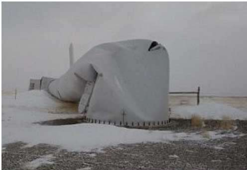
Wind Tower destroyed by Wind in Windy Wyoming
